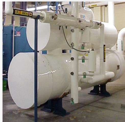
Shell-and-tube liquid chiller
