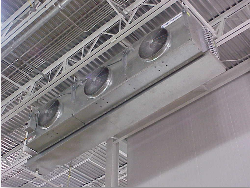
Ceiling-hung evaporator in a dock area
