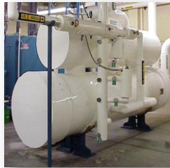
Shell-and-tube liquid chiller
