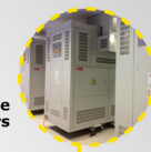
Scrubber Water Type VFD in ventilation fans to regulate the air flow
