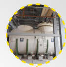
Scrubber Water Type VFD in ventilation fans to regulate the air flow
