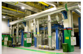
Evaporators Stainless Steel and Semi-Welded plate heat exchanger
