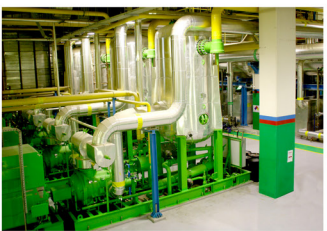
Compressor Units Taylor Made Chillers designed and fabricated in Araner's Workshop 2,500 TR Screw Compressor High efficiency and reliability
